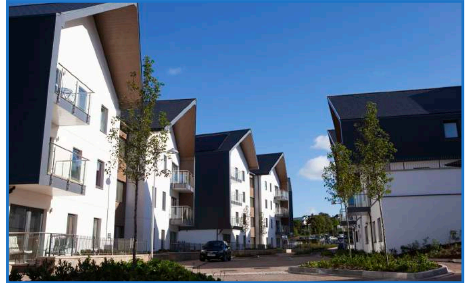
New housing development, Beechfield View, Torquay
